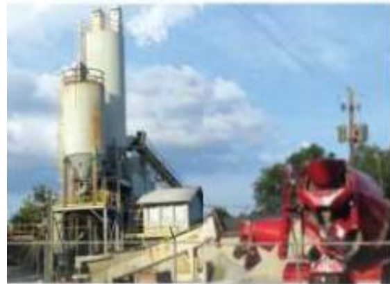
Fig.20- Cement Manufacturing Plant
