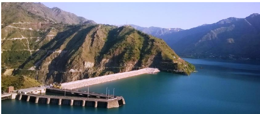
FIGURE 6: View of Kol –Dam reservoir after completion of project during 2014.
