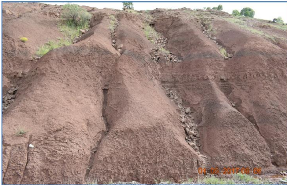
Picture 2: Water rill erosion on the slopes of the study area
